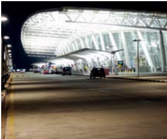
Chennai International Airport, India
